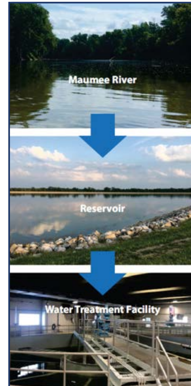
The City's Water Treatment Plant (WTP) draws water from the Maumee River to replenish its 74 acre upground reservoir which acts as a pre-treatment basin.
